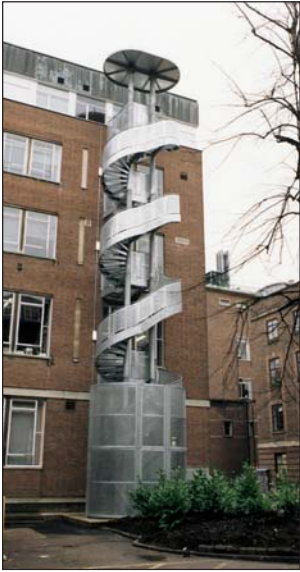
Spiral fire escape staircase with canopy and security cage.
